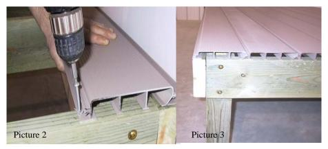
Install Deck Plank male flange into female starter strip, hold snug (self spacing), use #10 stainless steel fasteners at each joist to secure as shown in picture 2 Repeat until you reach the edge of the framing as in picture 3 Note: Should the last plank width be too great. Planking can be ripped to proper length with carbide saw blade using skill saw or table saw. The plank can then be fastened with a #10 Stainless steel fastener applied at an angle.
