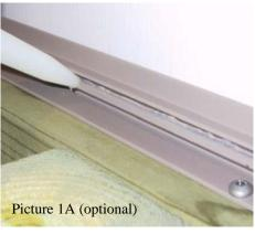
Optional Step: Apply clear silicone sealant (sold separately) in female groove as shown in picture 1A
