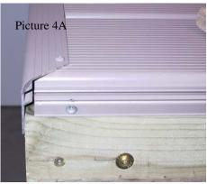
Edge Trim lengths allow 6" of extra material for miter cuts. Measure outside framing, for a typical 90 degree corner as shown in picture 4, adjust saw to 45 degree angle.
