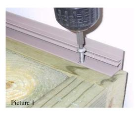
Hold *Starter Strip* next to house, Use #10 stainless steel fastener as shown in picture 1
